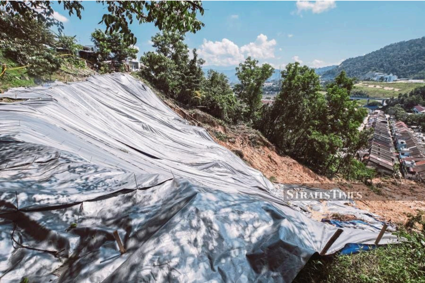
A canvas sheet cover is used to prevent soil erosion in a housing area. In extreme cases, soil erosion can cause building collapse. FILE PIC
