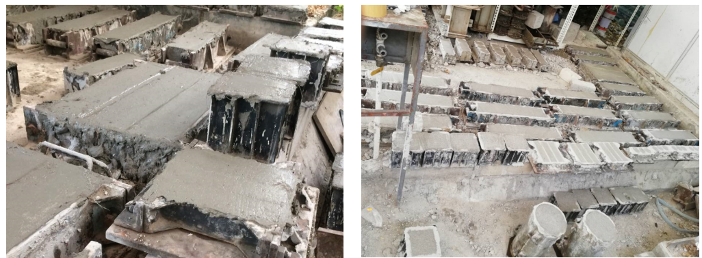
Figure 3. LFC slurry was then poured into molds.
